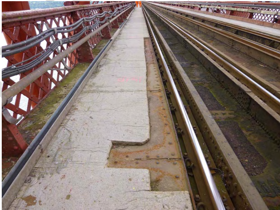
Typical condition of cess walkway
