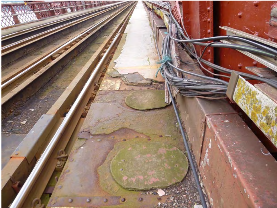
Cess walkway exposed steel and timber lids before preparation and coatings
